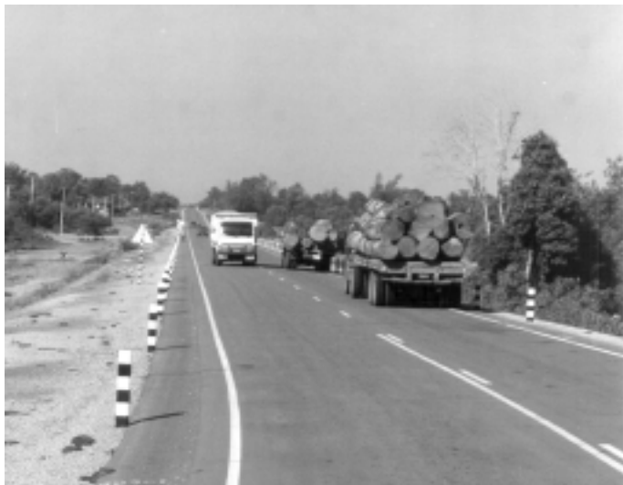
Route 9. The East West Corridor in Laos, a flagship GMS project promoting regional trade integration. (Source: Jonathan Cornford)
