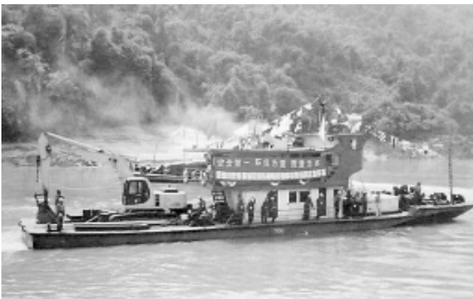
Chinese boat engaged in rapids blasting along the Mekong with the purpose of improving the shipping channel.
